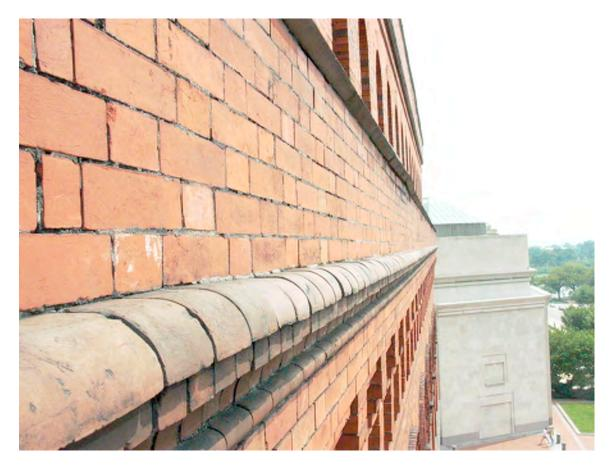
All stone and terracotta outcroppings or projections would do well to be capped in metal. Copper would profoundly stain. Lead-coated copper would not conform to the irregular masonry tops. Lead however is able both to fully conform to all irregularities in the surface below and has enough integral weight that additional attachment methods apart from letting the top edge into a mortar joint and setting with lead wedges would be unnecessary.
