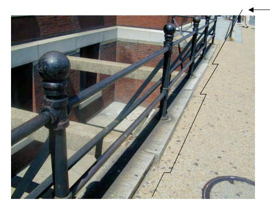
Buttressing concrete insets worsened misalignment stresses on moat retaining walls - both stone and brick
