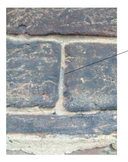
Scratching the white surface crust of an original joint reveals the dark bedding mortar below.
