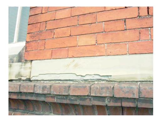
Stone failure due to stress fracture is most often seen in the granite elements that are very long compared to their thickness. This is particularly seen at window sills where the jambs are under a considerable load and the window area has almost none. The other stones seen as window sills show less breakage, likely because they will accommodate deformation better than the brittle granite. Where stone is stress fractured grout repairs would be appropriate.
